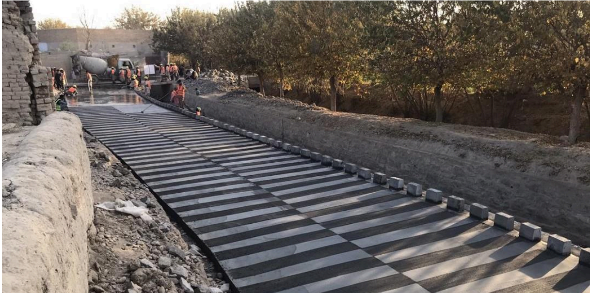
Street paving with plum concrete in project Construction of Fazli Plum Concrete Streets in District #6 of Kandahar city on 15 December 2024 by laborers
