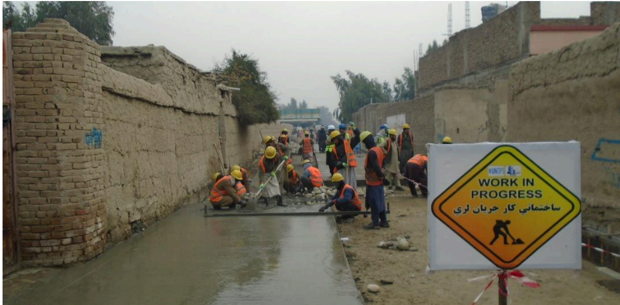
Street paving in project Construction of Plum Concrete Surface Streets of Wachtangi in Gozar# 40, District# 8, Jalalabad City on 23 December 2024.
